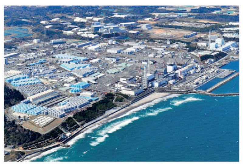
More than 1,000 tanks holding contaminated water are scattered around the site of the Fukushima Daiichi nuclear power plant in Okuma, Japan. Credit: The Asahi Shimbun via Getty
