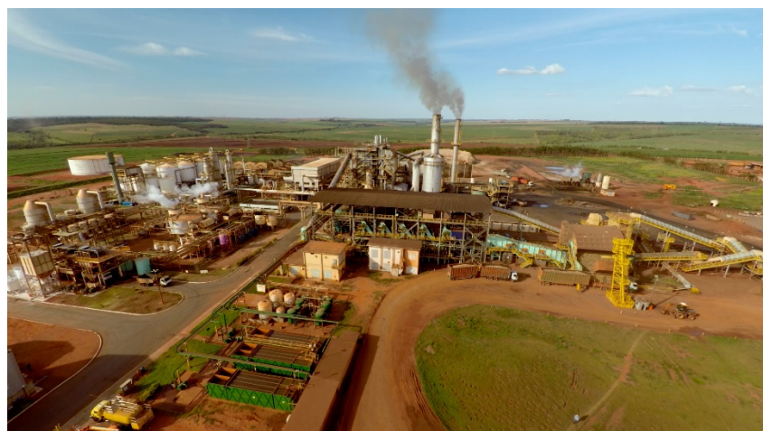
UMOE Bioenergy Plant in Brazil Photo: UMOE
